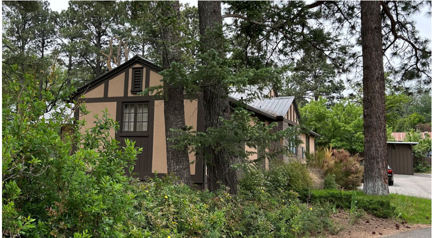
The Bethe House on Bathtub Row seen from the north.
